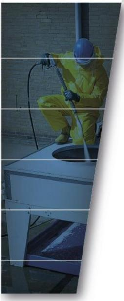
Cleaning and Coating Air-Cooled Heat Exchangers
