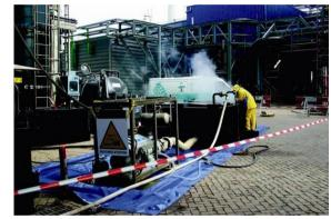
On-Line Cleaning of Furnaces, Energy Boilers and Incinerators
