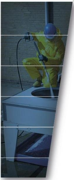
Cleaning, Disinfection and Renovation of Air Handling Units
